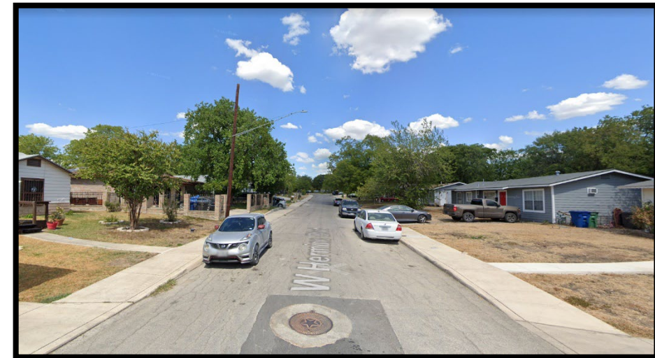
Hermine Blvd. MH #2559 (Facing East)
